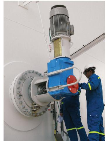
Swivel type mixers allow the mixer flow to cover the complete tank bottom with minimum power consumption. The mixer is selected to produce a flow that can reach the opposite side of the tank. By changing the angle monthly, the flow can be positioned to control BS&W in different sectors of the tank bottom. Planning a monthly angle change sequence allows you to avoid all deposits.
